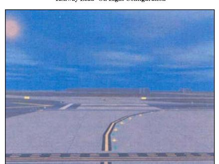
FIG 2-1-12 Taxiway Lead-On Light Configuration
